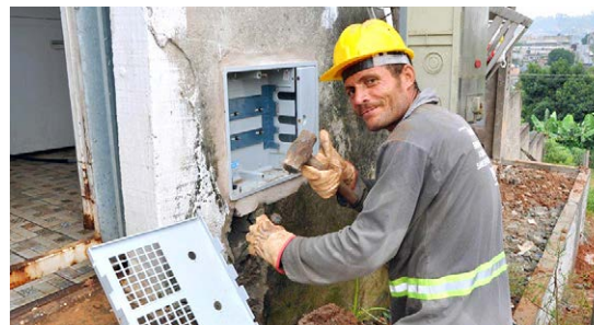
New water connection is completed in Itaquaquecetuba
